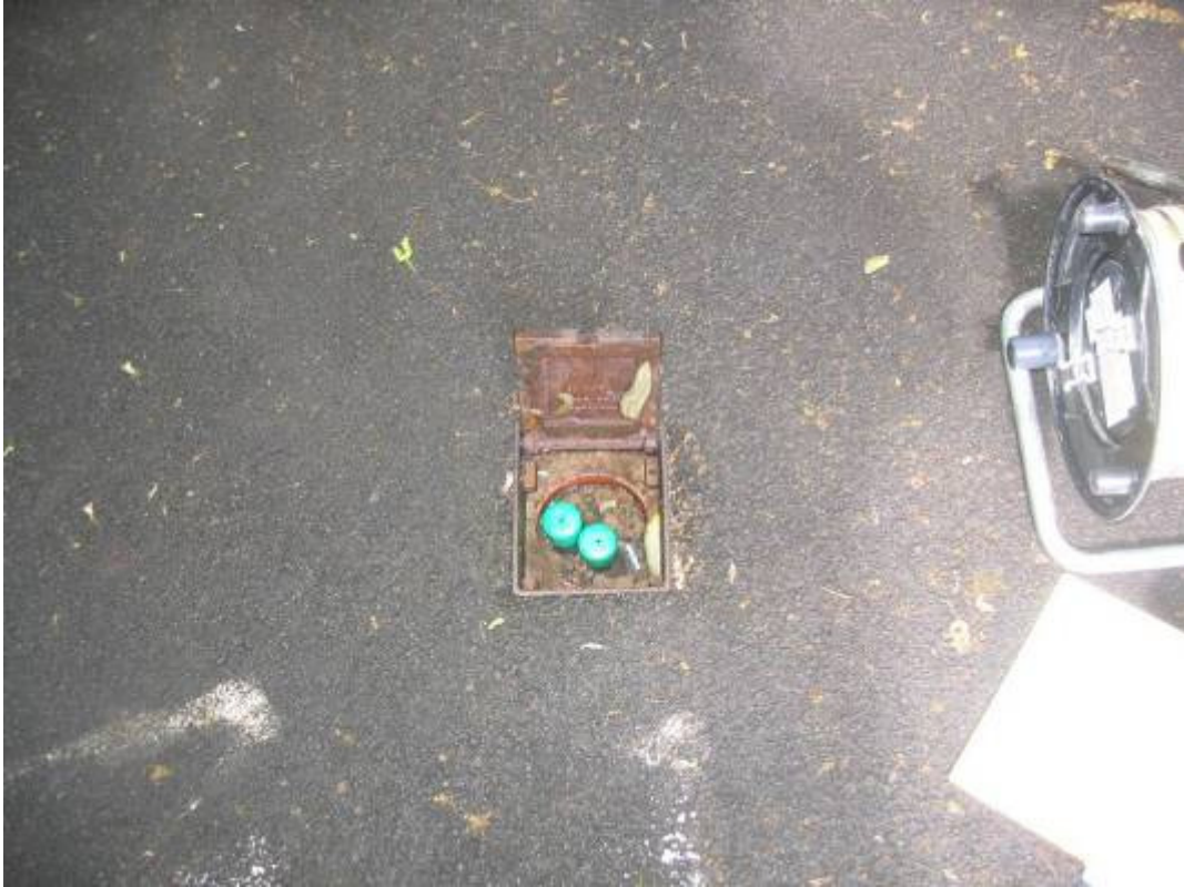
Plate 48 Scarborough South Cliff D2
