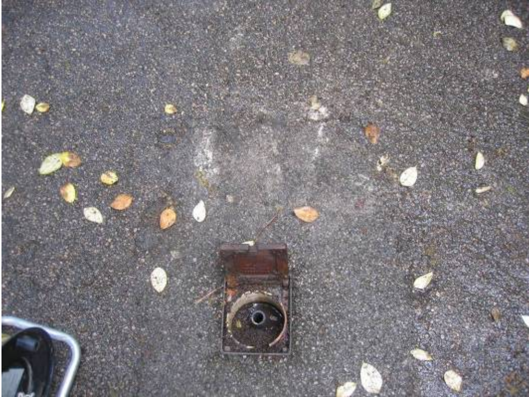
Plate 36 Scarborough South Cliff H5
