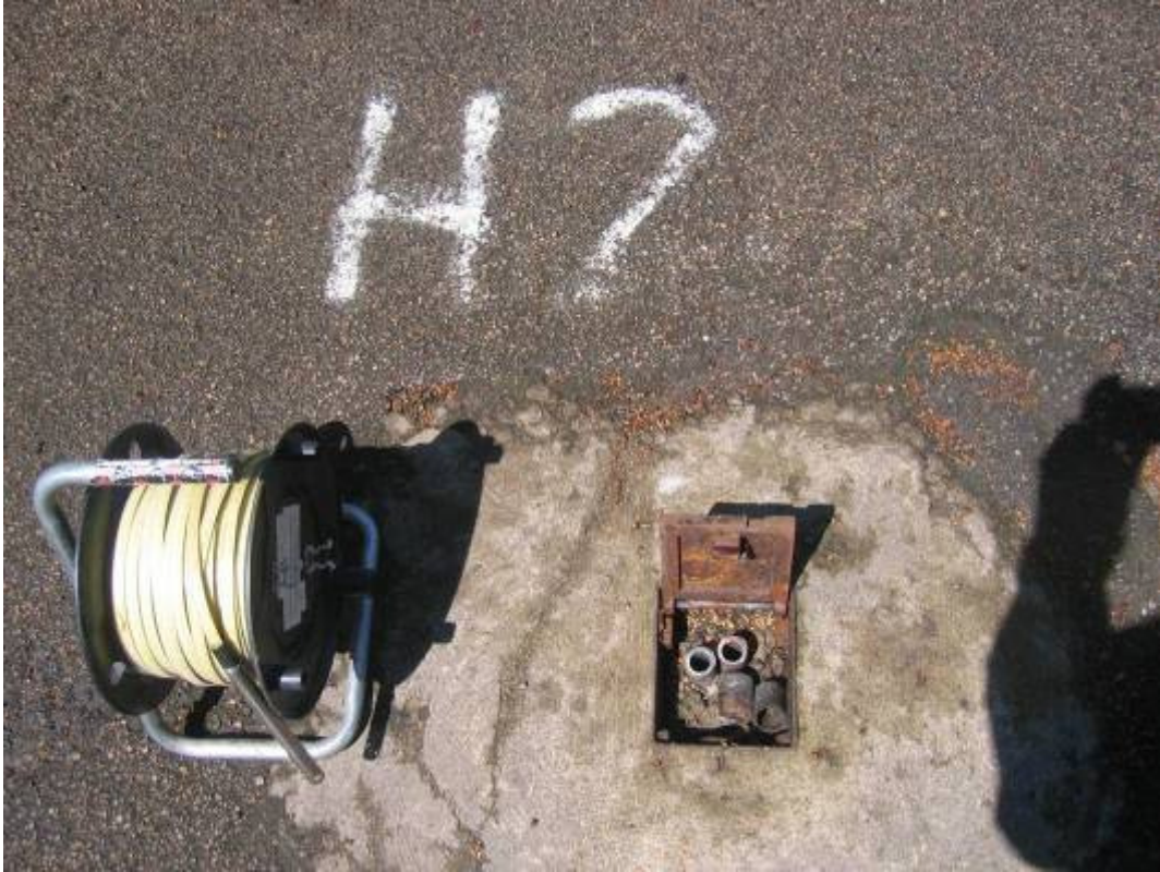
Plate 34 Scarborough South Cliff H2
